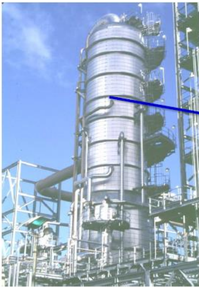
Distillation columns e.g., in petroleum refinery
