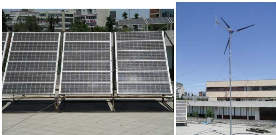
**Fig. 10.8** The hybrid energy system that powers the RO at the Agricultural University of Athens
