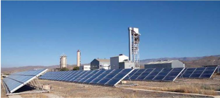
**Fig.10.1** The solar thermal field of the solar MED plant in Almeria
