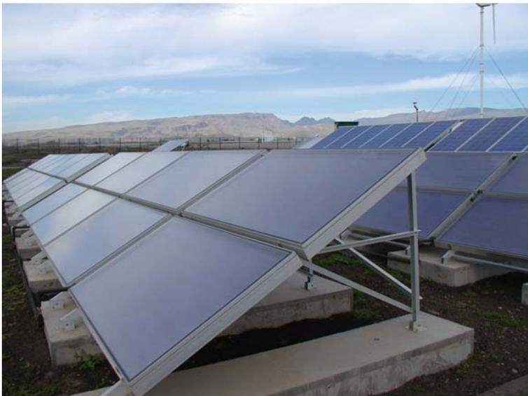
**Fig. 10.4** The solar collector system of the 1 m<sup>3</sup>/day MD plant
