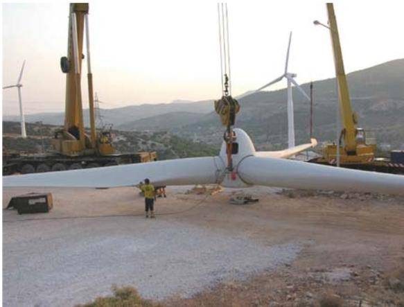
**Fig. 9.3** Erection of the rotor of a W/T
