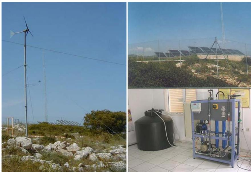
**Fig. 10.9** The hybrid RO system installed in Lavrio by the centre for renewable energy sources
