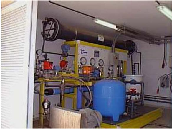
**Fig. 9.21** The RO unit at Pozo Izquierdo
