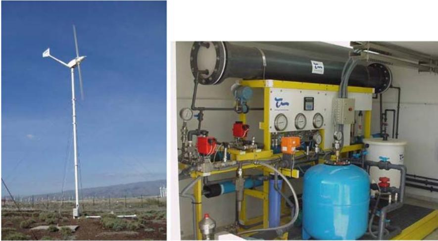
**Fig. 10.7** The ITC wind/RO system in the Canary Islands
