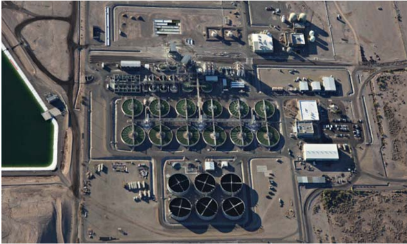
Figure 14.10 Palo Verde Water Treatment Plant (from Lott 2011).
