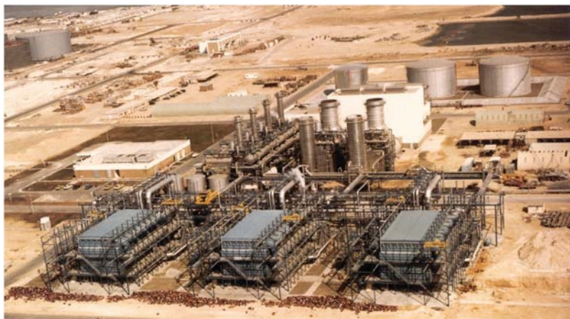
Figure 2.55 Umm al nar east electricity and water generation plant (by courtesy of Sidem)[14].
