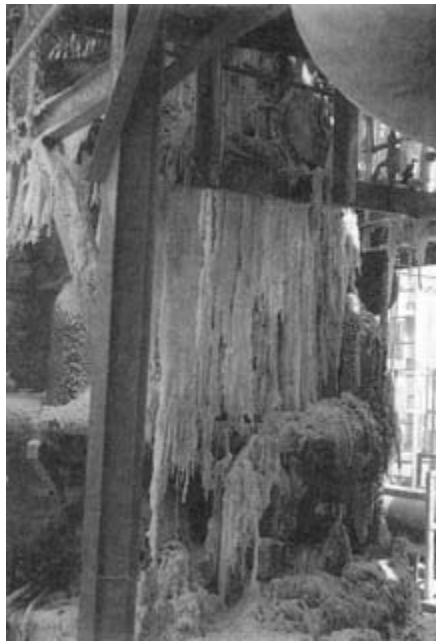
FIGURE 6-7 Icicles are formed from leaking caustic soda that dripped from an evaporator flange.
