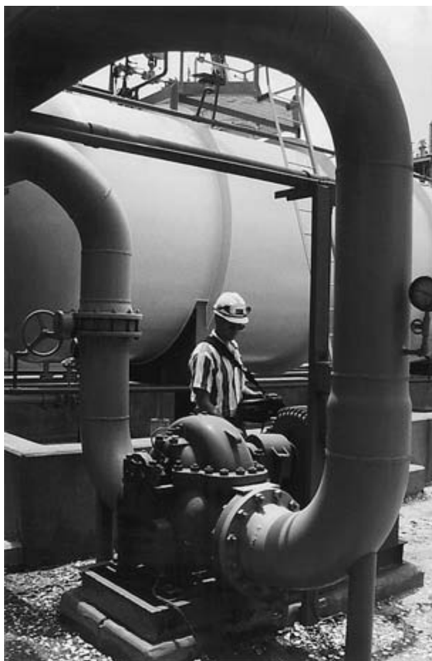
FIGURE 10-2 A vibration technician taking readings on a cooling water pump.
