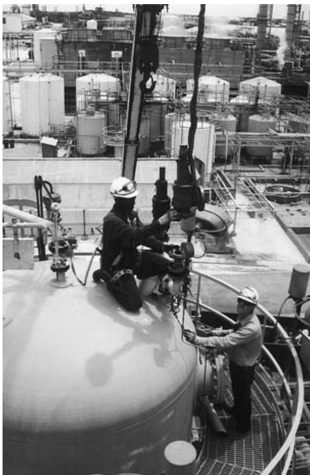
FIGURE 10-20 A mechanic is reinstalling an SRV after it was tested in the shop and raised into position by a crane.
