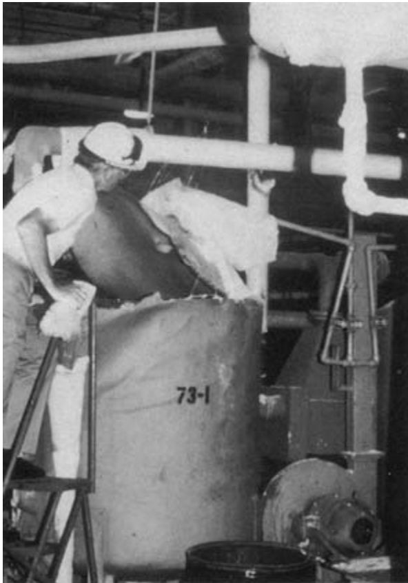
FIGURE 2-21 Employee examines the air dryer failure.
