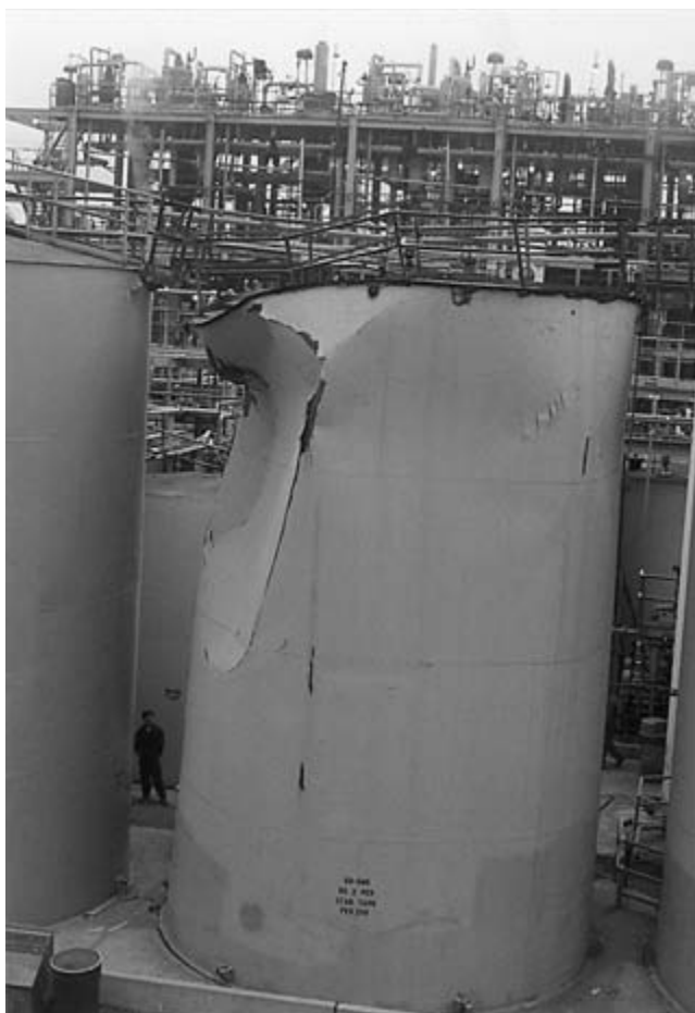
FIGURE 2-16 Crushed tank in the tank farm.
