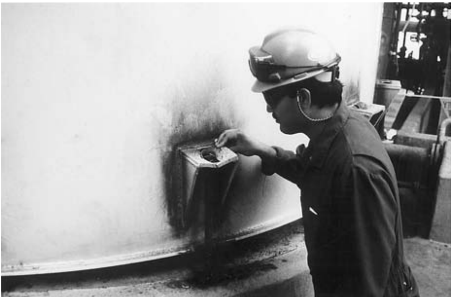
FIGURE 3-4 Tank bottom is bulged and anchor nuts are pulled through the anchor chairs.
