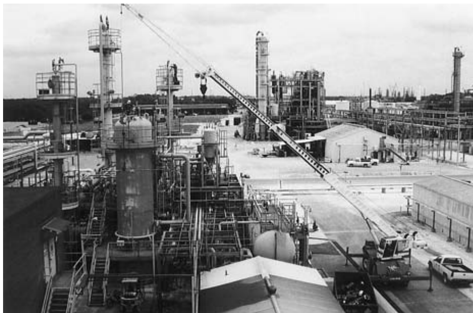
FIGURE 10-19 A crane is lifting a recently tested and reconditioned safety relief valve to reinstall on a reactor.
