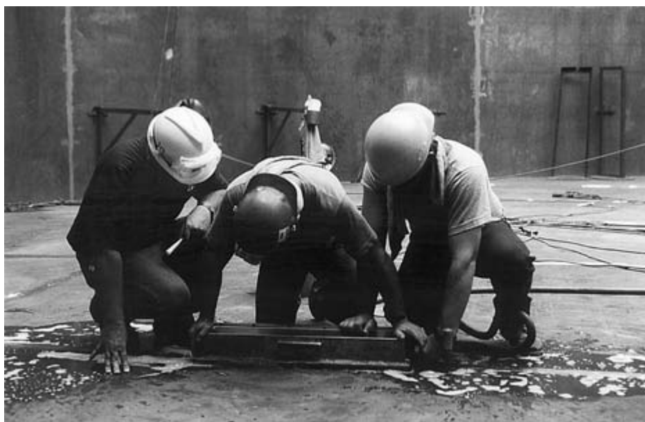
FIGURE 10-13 Inspectors using a vacuum box and soapy water to check for leaks in welds on the floor of low-pressure tanks.
