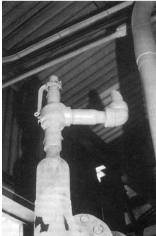
FIGURE 6-13 A threaded safety relief valve reinstalled with a reduced discharge piping arrangement.
