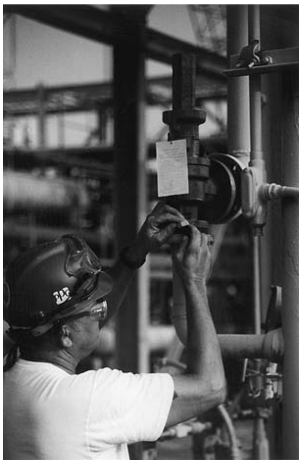
FIGURE 10-17 A mechanic is removing an SRV from a unit. The mechanic records the condition of the inlet and outlet piping components on the tag before the valve is sent for testing.
