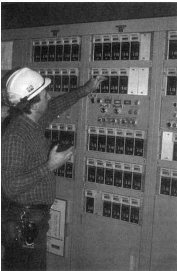
FIGURE 10-25 An instrument mechanic proof-tests a critical instrument panel.
