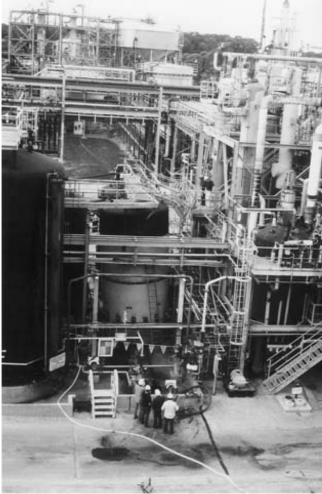
FIGURE 3-1 An API 620 tank is damaged during a hydrotest.
