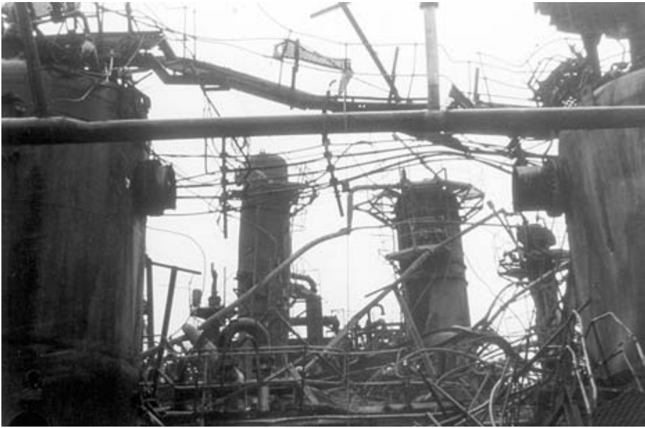
FIGURE 5-16 A Destroyed Section of the Flixborough Reactor System. Photo courtesy of Trevor A. Kletz.
