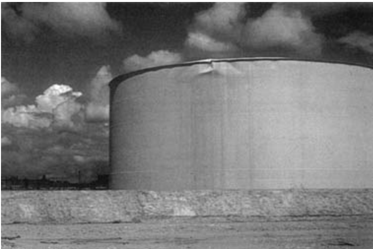
FIGURE 2–12 Large tank (100-ft. diameter) damaged by overfilling.
