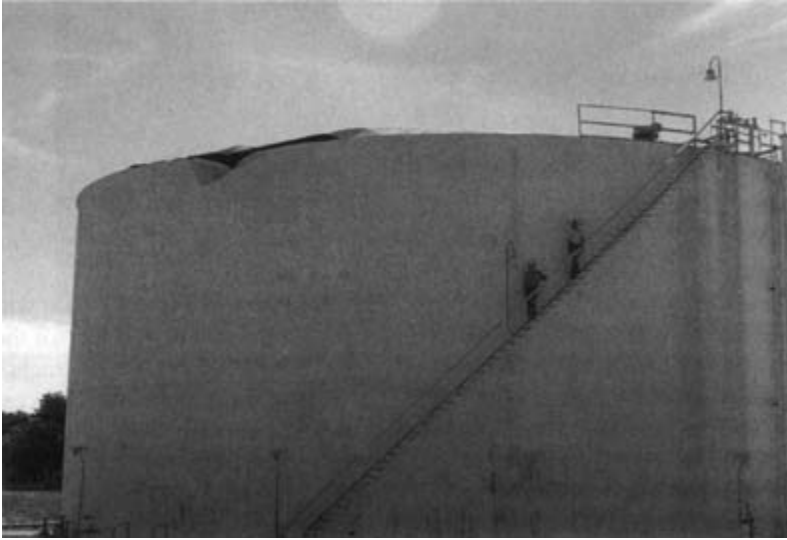
FIGURE 6-11 Overpressure problems created by a one-minute modification and changing weather.
