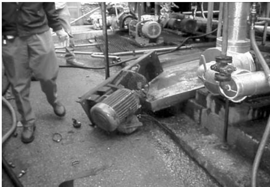
FIGURE 7-13 Pump base plate and motor thrust into walkway. Courtesy of Eastman Chemical Company.
