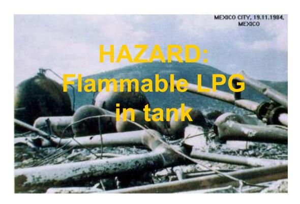
LPG explosion caused by a leak at a marketing terminal pipeline that ignited and started a fire at the terminal.
