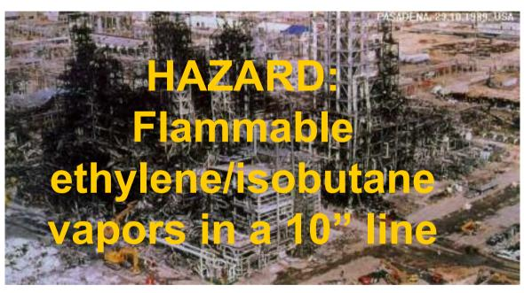
A seal blew out on an ethylene loop reactor, releasing ethyleneisobutane vapor cloud, a compound used in making plastics
