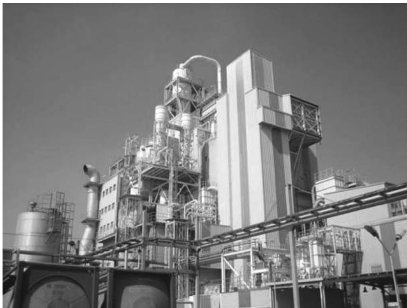
FIGURE 19.7 A typical manufacturing unit for spray dried detergent powders.
